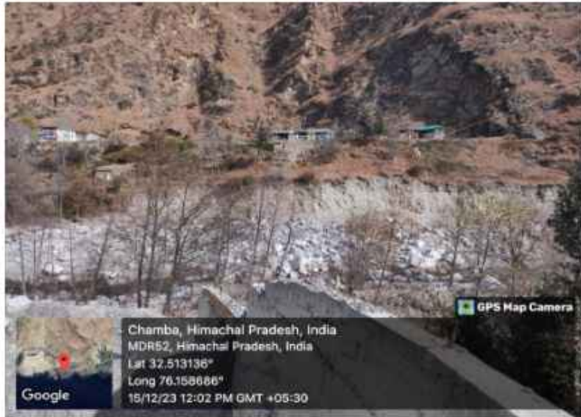
Fig.40 Image depicts river erosion at Village Saloon long Holi road.
