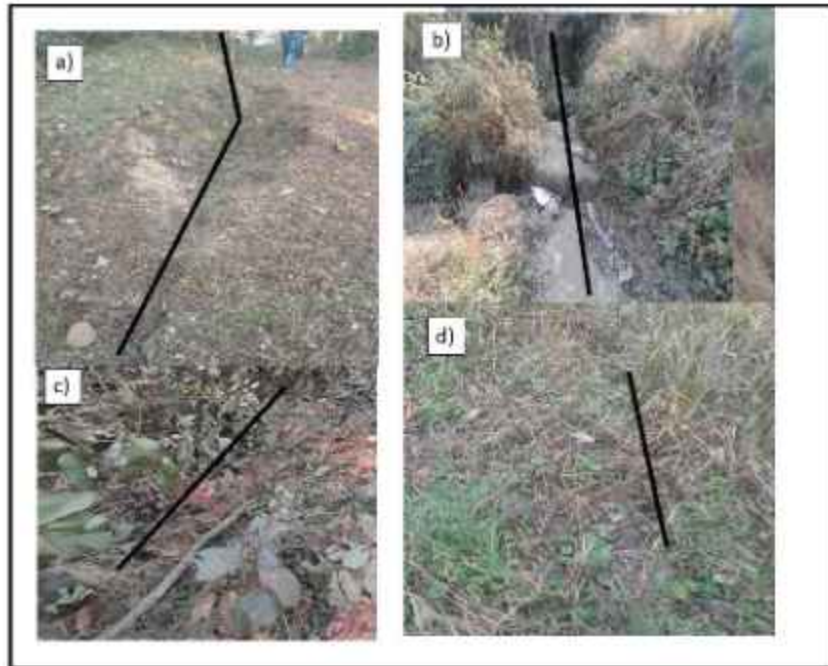
Fig.28 a, c ) Shows the development of land fissure and its direction at the summit of the landslide zone Images b) indicated the natural drainage present in the same summit zone by running along the slope direction. d) Again showing the direction of the fissure developed in the upper part of the slide zone.
