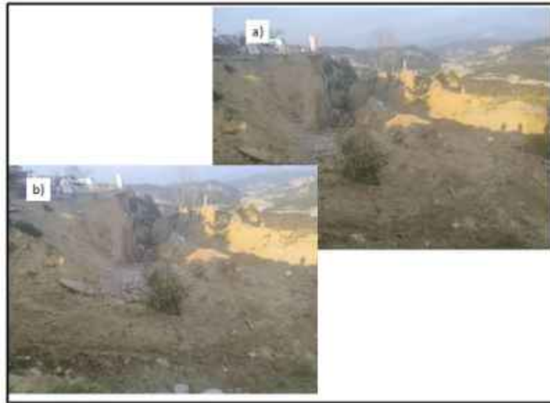
Fig. 15 Sandstone rocks get displaced along the fissure and caused disastrous impact in the village. All houses located on this portion of the sheet like rock also displaced.
