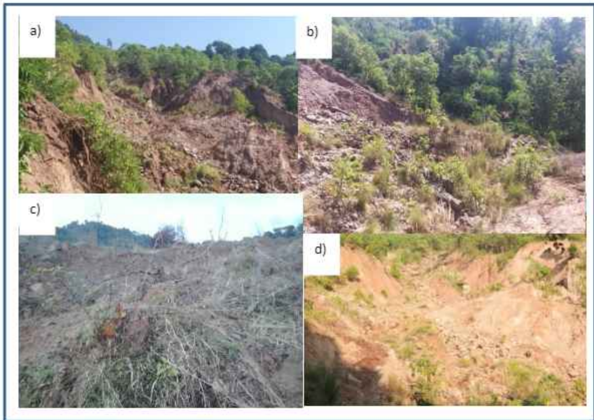
Fig. 19 Shows lithological characteristics of the slide zone: a) The area on the left of the slide zone, which was exposed due to the activity in the region; b) shows the presence of weathered rock material from the scarp region; c) the central part of the slide zones in the western side indicating weathered soil with uprooted trees and bushes, d) uneven topography on the southeast part of the slide in the slide zone with sandy to fine soil particles.
