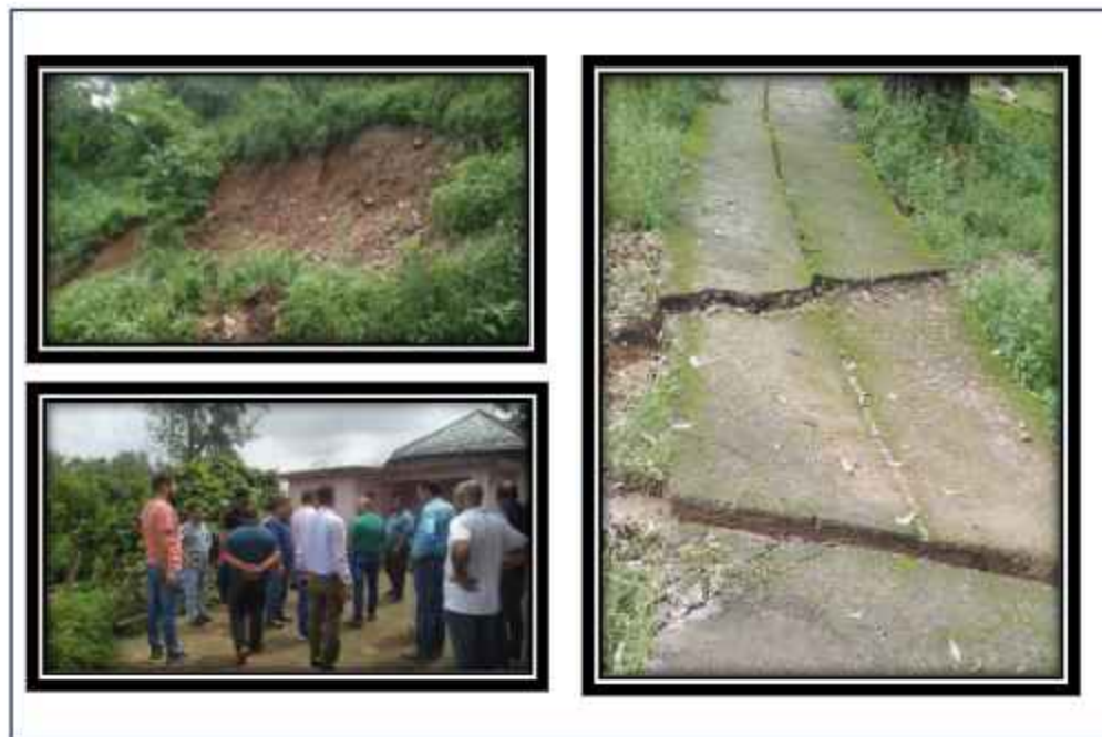
Fig. 7 Shows the scarp in the second slide zones and house with in the slide zone.
